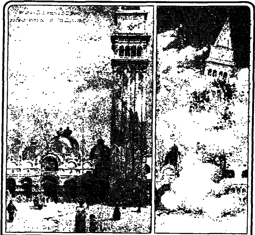
Postcards depicting the 1902 collapse of the Campanile of St. Mark's.
